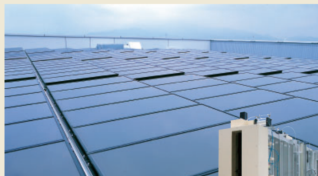
The solar panels set on the roof of the Chigasaki Factory
