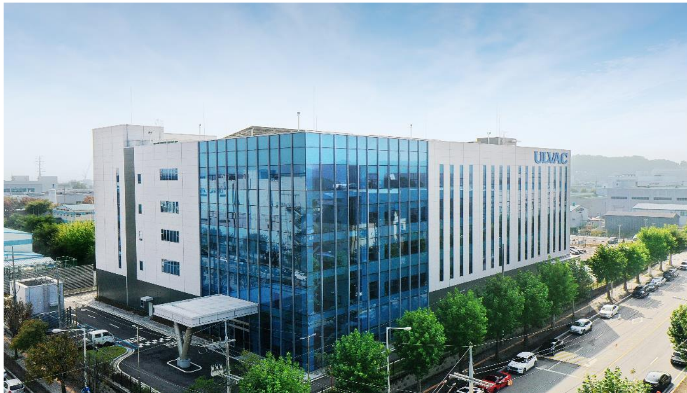
Technology Center PYEONGTAEK, Pyeongtaek, Korea
